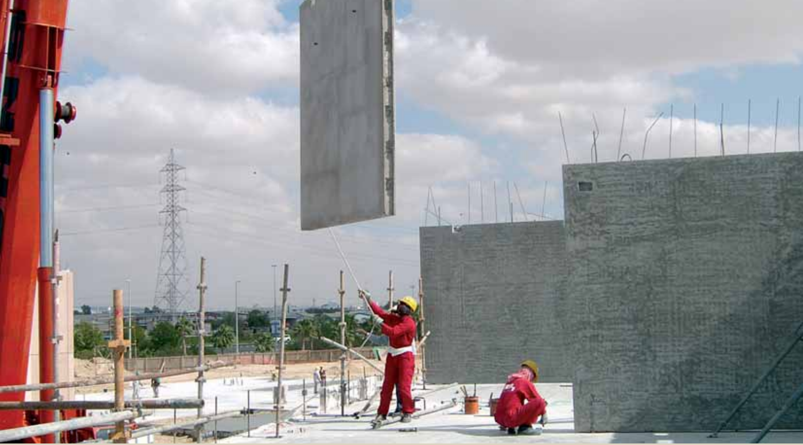
The plant in Abu Dhabi has delivered columns, beams, stairs and internal walls for American School. Here wall panels are erected.
