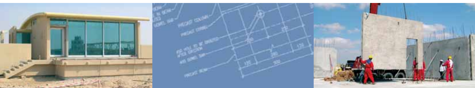
In Dubai the precast concrete elements for a number of VIP Guest Villas have been erected.
